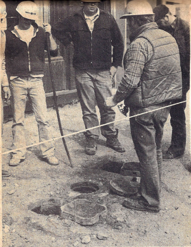
GAS MAIN REPAIRED - When the sidewalk along Main Street in Adams collapsed last Wednesday, natural gas began spewing from a ruptured main. Niagara Mohawk workmen quickly turned off the supply to several businesses and began making repairs to restore service. Several businesses along the street were temporarily evacuated due to the strong odor of gas. Service was restored to most customers in a few hours, but businesses over the creek remained without service until an alternate line could be installed.
